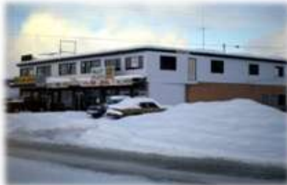
Atwater building in Eagle River – the church met upstairs,
